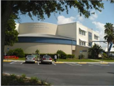
Exterior Stucco Repair and Repainting
